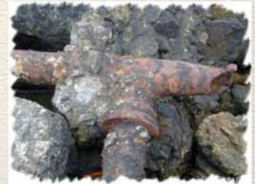
THESE PIPES ARE IN THE MIDDLE OF CHEMICAL CHANGES AS THEY RUST.
